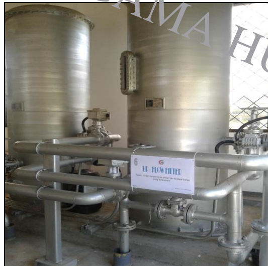
Gambar 5.8 Up Flow Filter IPAL RSUD dr. H. Koesnadi Bondowoso (2023)
